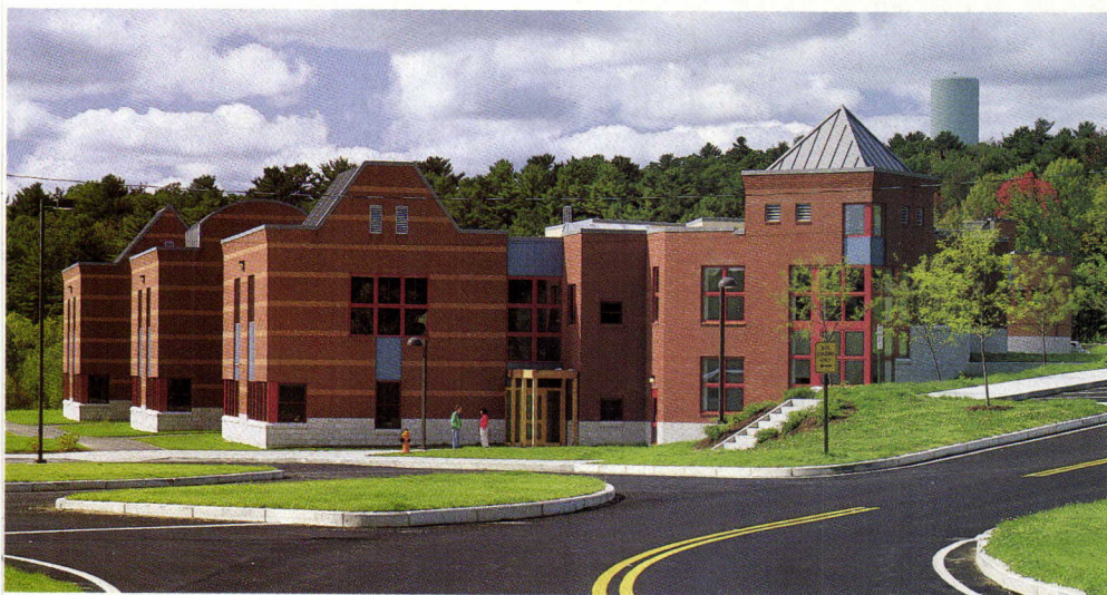
Honorable Mention Mast Landing School (above) Freeport, Maine Stephen Blatt Architects
