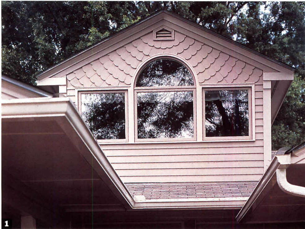
1. Sharon Harris of Pro Designs in Raleigh, North Carolina, used Fancy Cuts shingles of western red cedar. Shakertown. Circle 402 on information card
