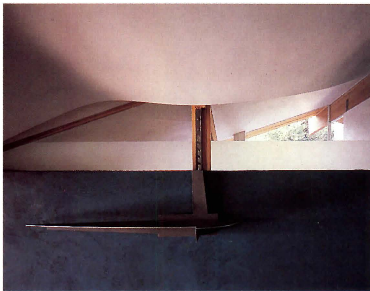
Barragan meets Schindler, Neutra, and Gehry with a twist in Frank Israel's radical renovation of a 1950s tract bungalow on the upper slopes of Beverly Hills (previous pages). Two views of the junction of the metal roof and zinc-clad walls reveal the glazing of the west-facing study (facing page, top) and bathroom wing with glass blocks set into the corner of the living room (facing page, bottom). In the bedroom, a Neoconstructivist canopy suggests a traditional four-poster (top) set off by curving burgundy plywood screens around the fireplace and in the headboard. The entryway (above) is defined by an undulating ceiling, a dark stucco wall, and a knife-edged metal shelf. Axonometric (below) shows the two-level rectangles that comprise the plan, with low-sloped roofs linked by a central trough.
