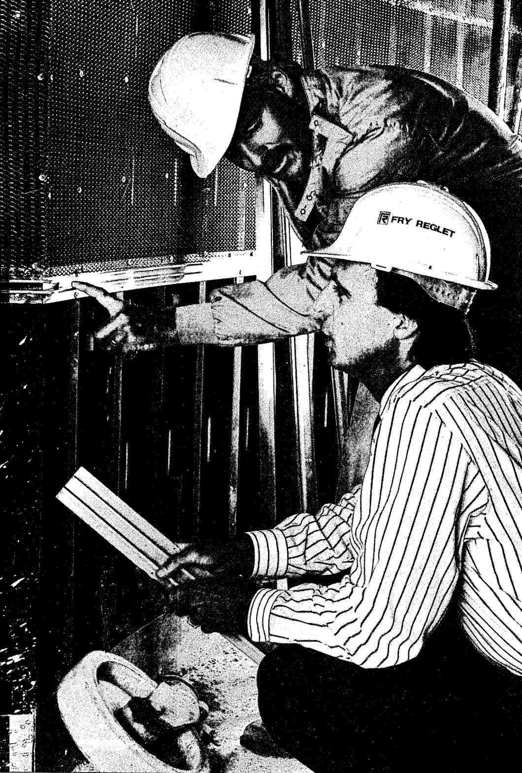
Fry representative consults on site of Library Tower project, Los Angeles, California. I.M. Pei & Partners, Design Architect. Ellerbe Becket, Executive Architect.
