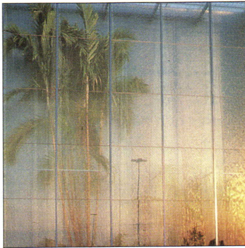
Left, the Best showroom in Hialeah, Fla., completed in 1979, has native vegetation enclosed behind a glass water wall.
