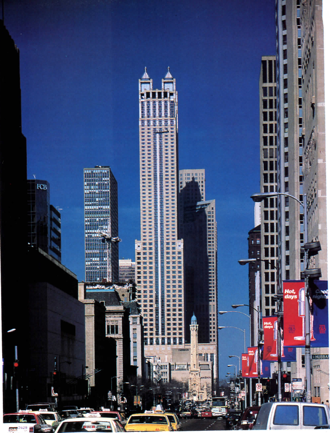
KPF's 900 Michigan Ave. building in Chicago, one of the newest composite structures. The section, left, shows flat slab construction for the top 30 residential floors. At the 30th floor, the load transfers to the steel frame of the offices, down to the seventh floor (retail), where the grid shifts again. The detail above shows the connection of concrete to steel.
