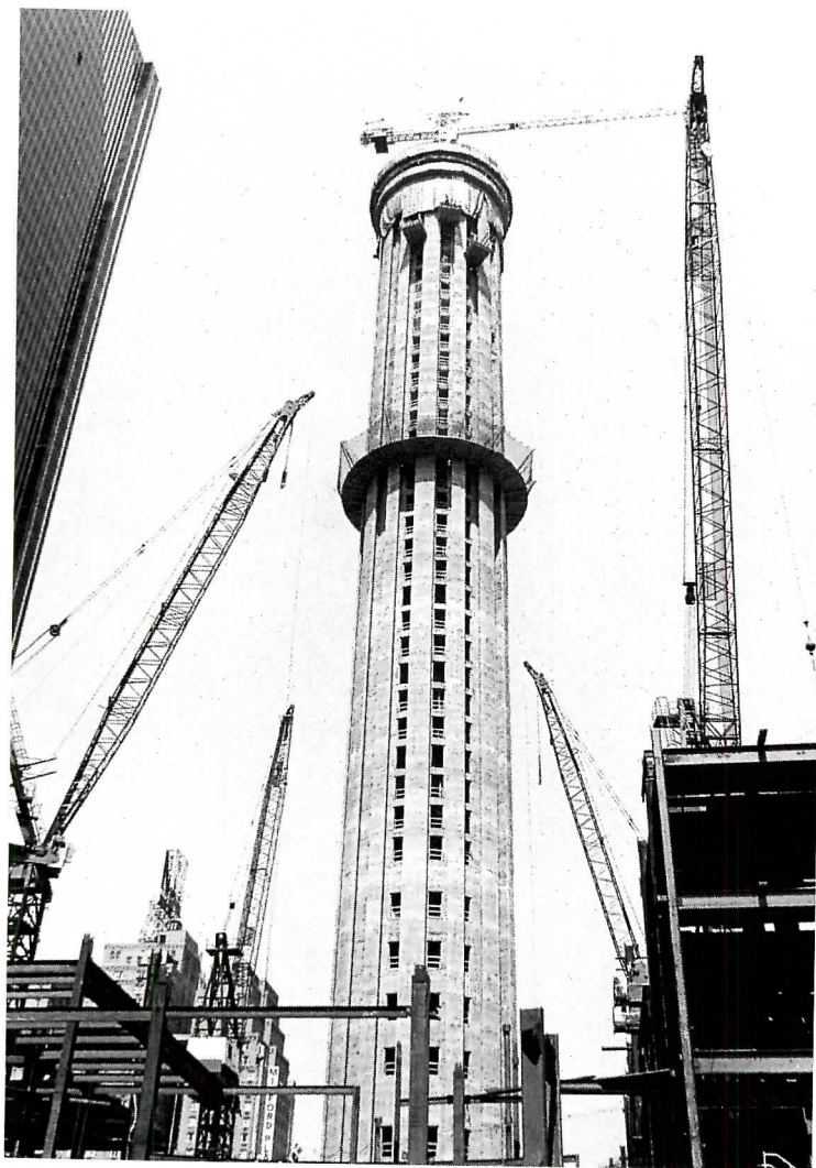
New York's Marriott Marquis, a tube frame above a braced frame.
