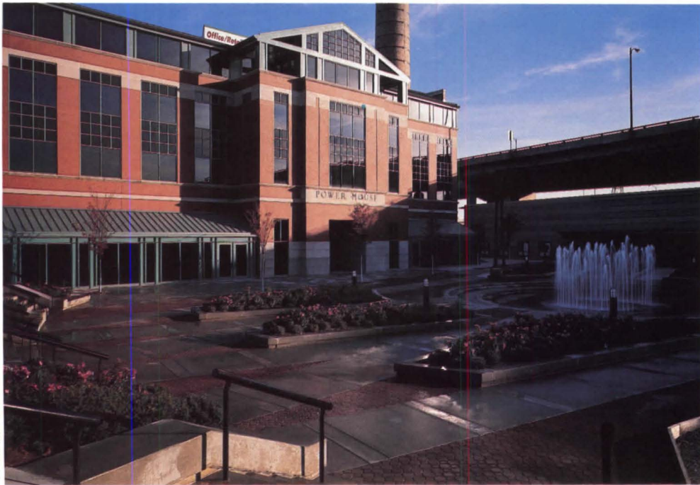
Left, a new Mackey Associates building on the foundation of an old powerhouse. The original smokestack remains. Behind the new building in the photo below is an old postal annex, restored and converted by Mackey. Facing page, two views of the restored shed. Bottom photo shows the low-keyed new hotel.
