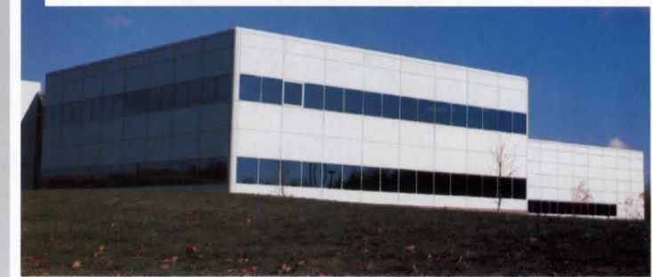
Siemens Corporation, Princeton, NJ Architect: Bowers Design Associates Princeton, NJ
