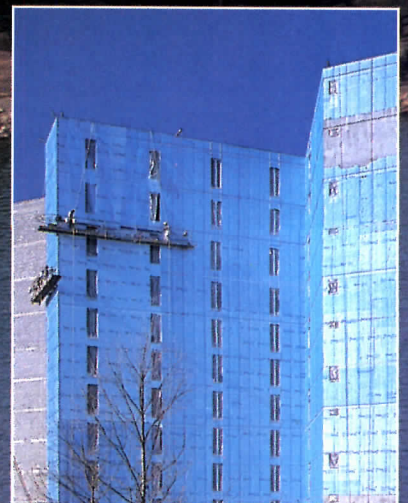
FULTON COUNTY JAIL, Fulton County, Georgia Now under construction Ova, Daniels, Busby — Architects
