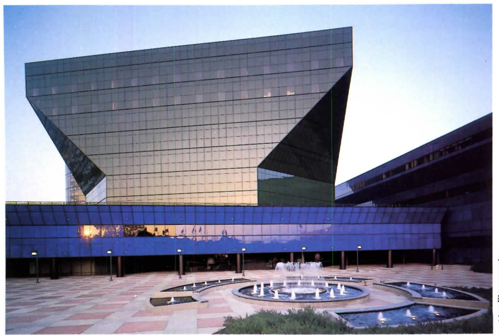
Above, the recent addition to Pelli's 1975 Pacific Design Center in Los Angeles. 'The Blue Whale,' as the 750,000-square-foot original has been dubbed, is tightly wrapped in opaque ceramic glass. The 475,000-square-foot expansion, sheathed in green glass, connects to the Blue Whale via a blue, story-high plinth. Another phase, yet to be built, includes a wedge-shaped red building.
