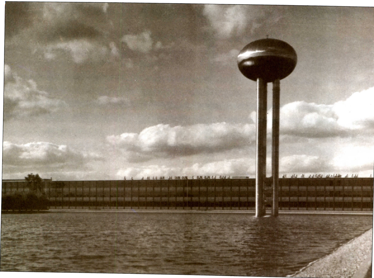
Left, steel frame of Burnham & Root's Reliance Building of 1894, one of Chicago's first skyscrapers; above, Eero Saarinen's General Motors Technical Center in Warren, Mich., was a testing ground for many building 'firsts.'
