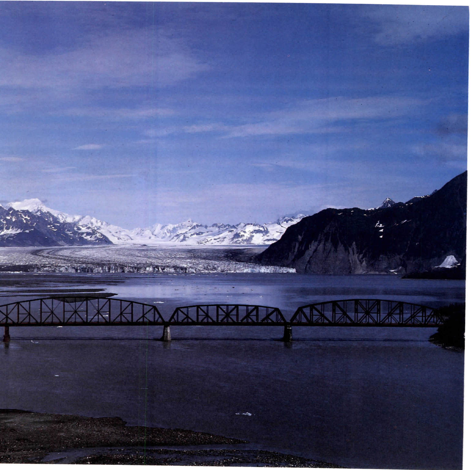
Top left, locomotive remains near Nome, Alaska. Above left, steam powered gas pumping station, Burnsville, W.Va. Above, earthquake damaged bridge in Alaska.
