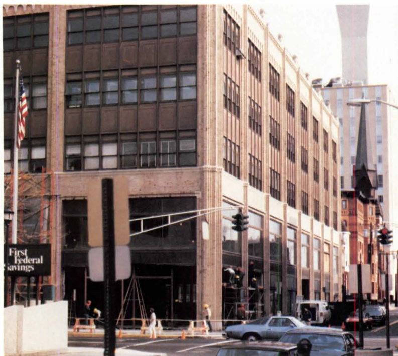
Below, before view of Orange Street facade of Roth & Moore's New Haven office rehab with tin infill, replaced with brick, in after view of Elm Street facade with new entrance (above). Projecting arms at building's midsection contain sodium vapor lamps that illuminate building at night.
