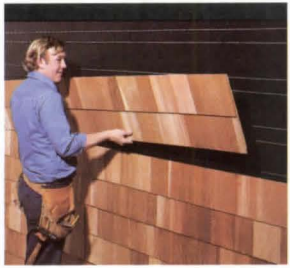
Install 8-feet of shingles in a shake.
