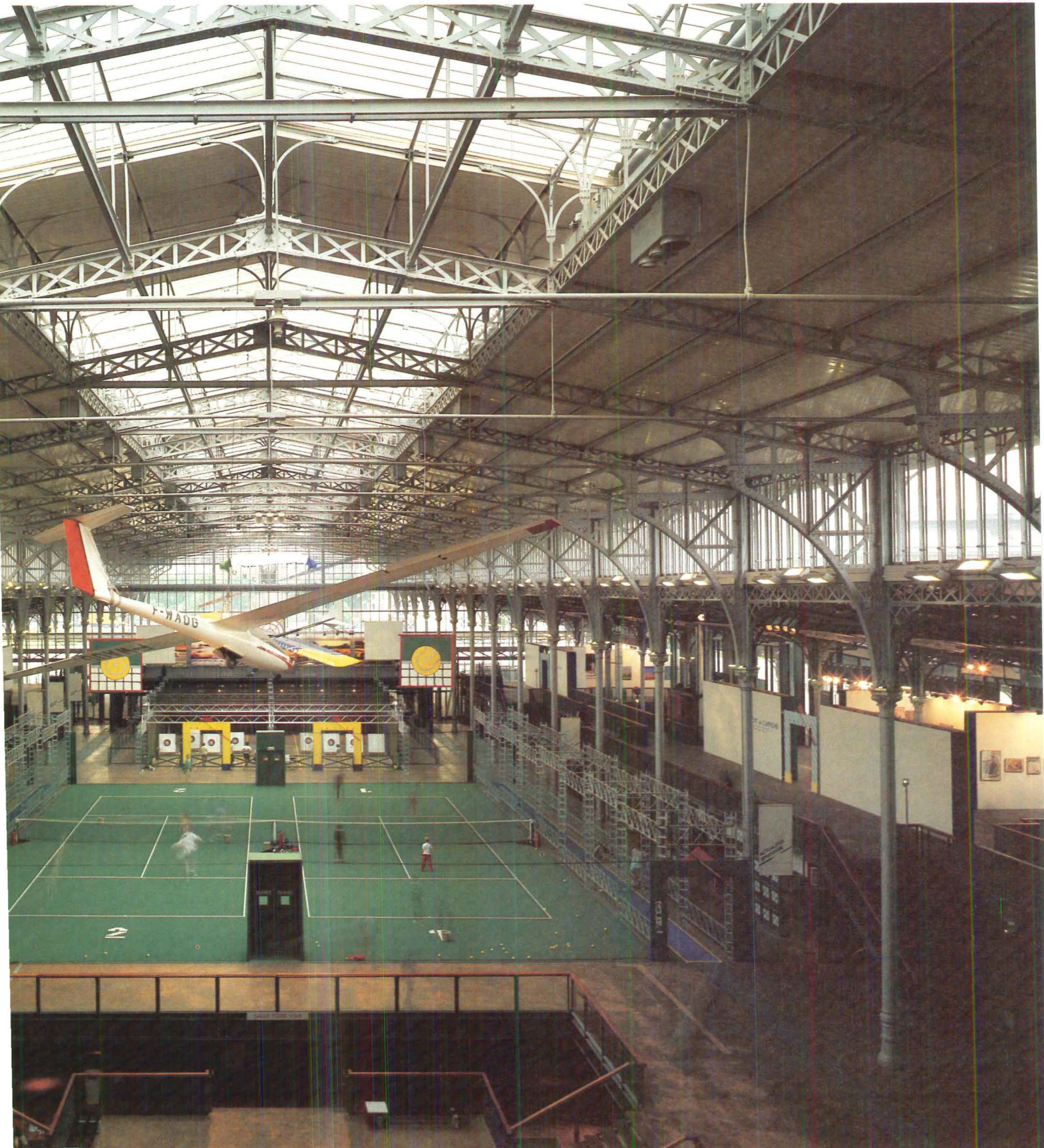
airy elegance of the 125-year-old Les Halles des Boeufs pavilion has been preserved and enhanced by a discreet intervention.
