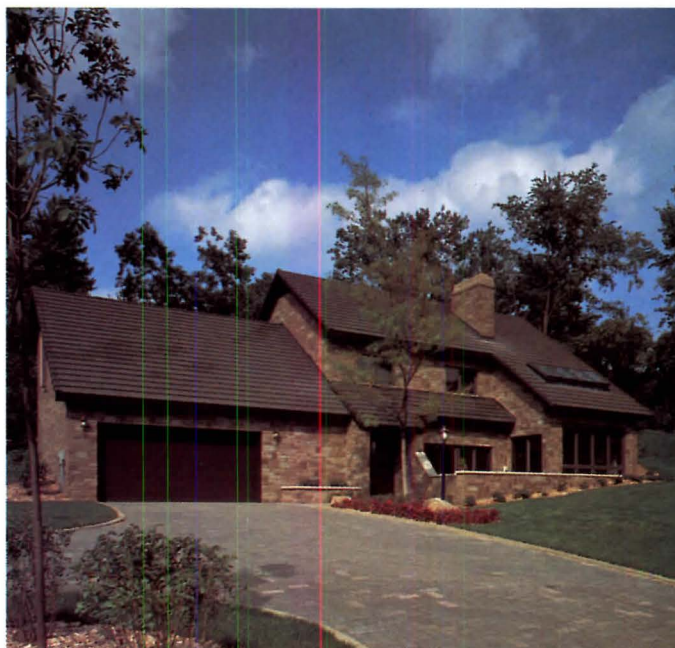
Shake style concrete roof tile system on a home in Minneapolis, Minnesota.
