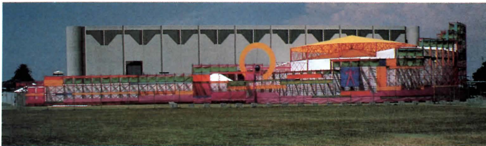
Summer Olympics Revisited: Located at Loyola Marymount University, the weightlifting pavilion was the first Olympic structure to use scaffolding. Because it was economical and could be used in a variety of ways, scaffolding was to become a major unifying design element among temporary Olympic structures (see Sept., page 51). Designed by John Aleksich Associates, the scaffolding and tented structure added 8,000 square feet to the university's athletic facility. It is basically an 80-foot-diameter drum made of a two-layer space frame. The tent canvases pick up the bright Olympic palette.
