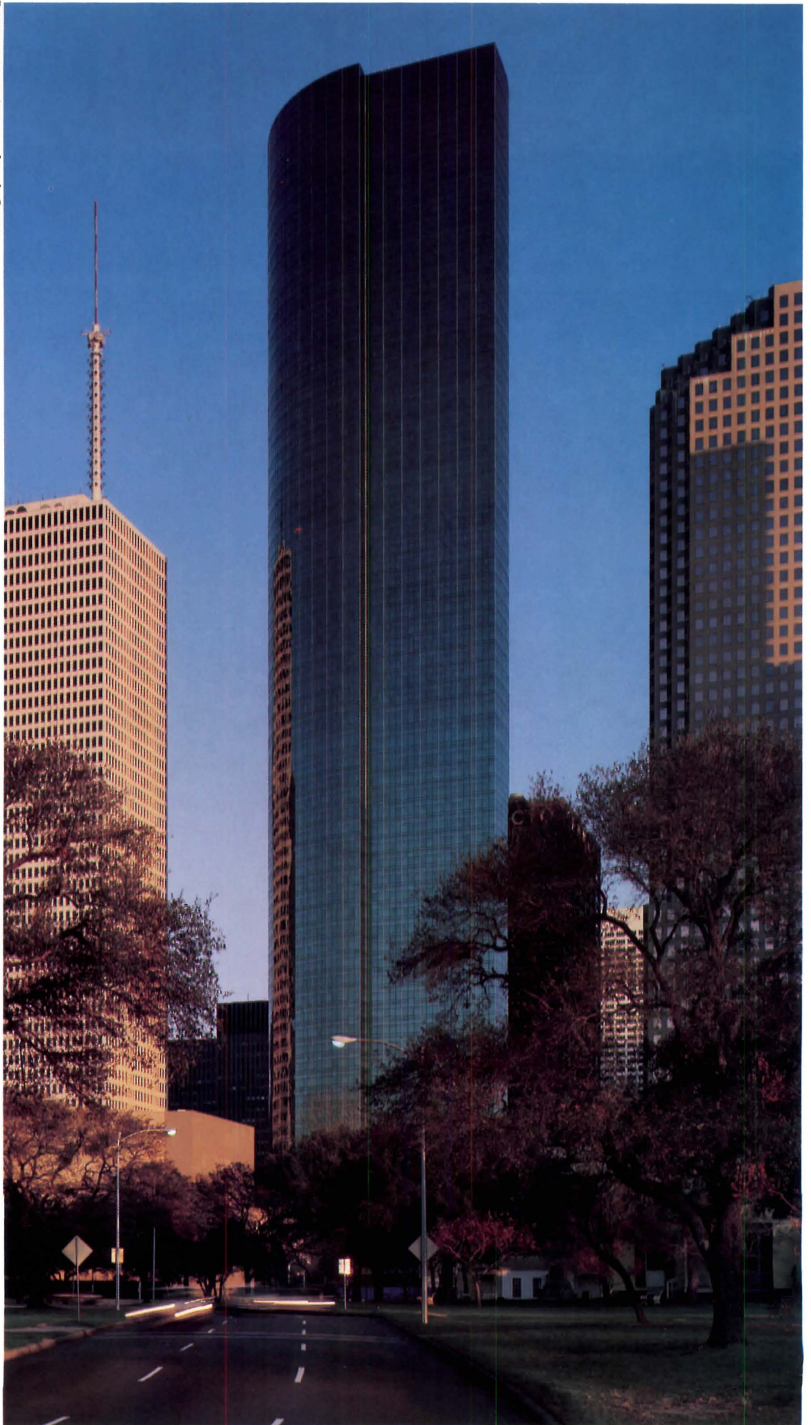
Allied, right, flanked by the travertine-covered Shell and sawtooth-topped Interfirst. Across page, Allied's polished granite base and a rendering of its glass skin from the inside.
