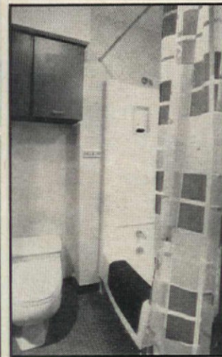
This view of children's bath (above) shows one-piece molded fiber-glass tub and shower unit that is not only extremely easy to install, but also a breeze to clean. Look closely at our "100-Plus Idea House" floor plans (next page) to see how the two compartmented baths have been planned and situated to serve individual family members as well as guests.
