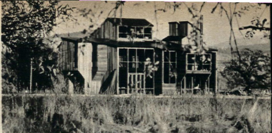
This house, built from 71-year-old redwood barrels, is a gem of shed-roof design.
