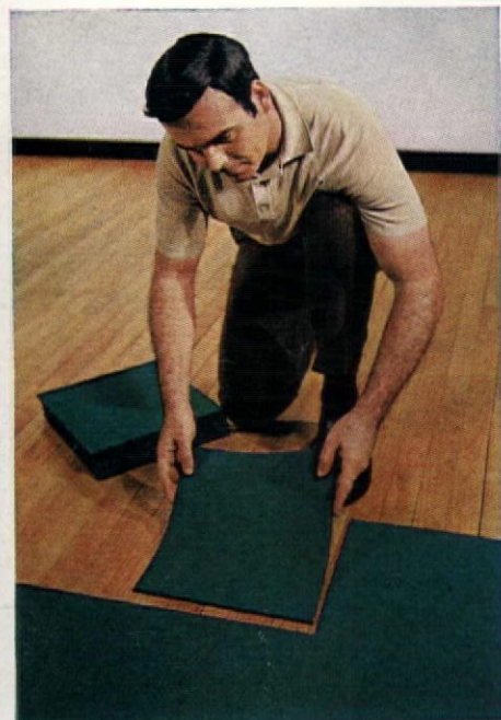
You can't make a mistake. If you install a tile improperly, just peel it up, reposition it, and press in place.
