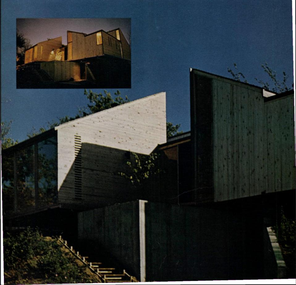
Ventilation slots were created by omitting every other board in parts of wall. (The large glass windows are fixed.) Vents are screened inside. A shutter opens for air flow. Walls are of cedar, an excellent insulator, and were left to weather, without any finish.
