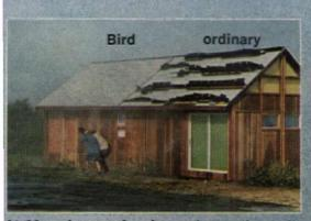
At 90 mph, over hurricane force, the ordinary shingles are flapping freely. Water begins to seep through the roof. But Bird Wind Seal JETS remain tight. Why? Because there are powerful, thermo-plastic dots on every Wind Seal JET - over 19,000 on an average roof. These adhesive dots weld the shingles to each other and to the roof. So even 120 mph winds didn't pry Wind Seal JETS loose.
