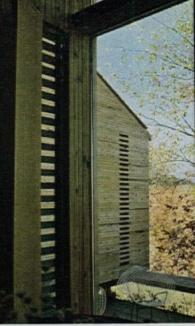
Living room (above) looks out to quiet countryside, has "paneled" walls of the cedar 2x2 construction. Detail (right) shows shutter that swings over slotted vent when not in use. Glass window is fixed. Wooden door to large deck outside dining room is nearby.
