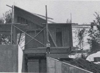
House under construction shows lumber strewn like spaghetti (top left) waiting to be nailed into place. At right is detail of corner, with two opposing layers of cedar 2x2s in wall interlocking with 2x4s of floor, to form extremely rigid, almost solid wood slab. Finished walls (directly above) are thus in place as house itself takes shape—no frame-it-then-cover-it sequence.
