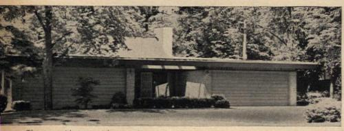
The street-side garage (above) is disguised to blend in with the overall design. The four-section overhead door on right wing is sided with lapped redwood to match bedroom wing, left.
