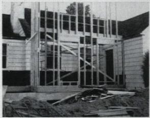
The before photo (immediately above) shows work in progress as the framing is roughed in for the addition at front and added second story. By comparing it with the after picture (top) you notice that the main entrance was moved from the extension at the right side of the house to the wing at the other side. Main front wall was moved forward.
