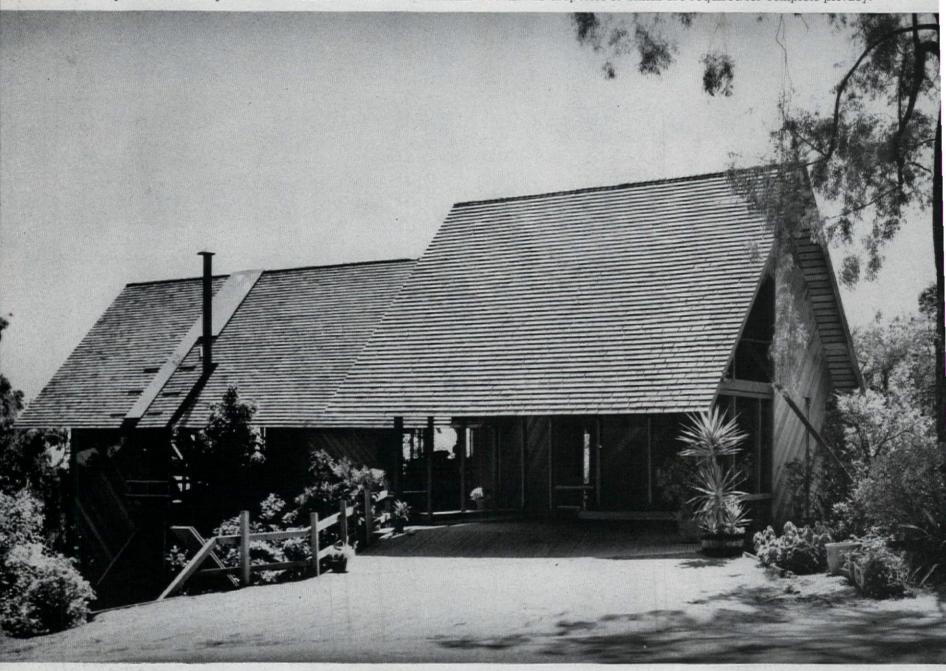
The middle floor of house (above) is on a level with the top of the ravine and is connected to solid land by the drive-way and entry deck. Main wing of house behind carport is supported on stilts in middle of the ravine. Concrete piles (right) supporting house have whirled lines left from cardboard pouring forms. The wooden joists, posts, and trusses are left exposed and are incorporated as an important visual element of design.
