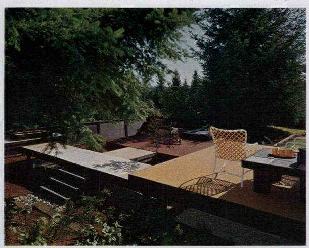
Besides the unusual design, this deck in Tacoma, Washington, is a departure from the usual spaced-board construction. Here, in this innovation by the American Plywood Association, it is simply a series of platforms of exterior-grade plywood, protected by plastic-based roofing material, set on the framing of 2x8s. On top of them is Ozite's Town 'n' Terrace indoor-outdoor carpeting, which is unaffected by rain and can be easily vacuum cleaned.
