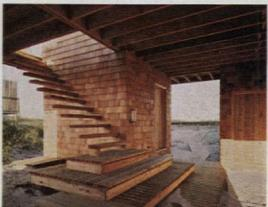
Exterior of house is a combination of the closed-in and the opened-up. Living room is in wide-windowed section between the towers. House has the locust-post foundation system typically used in the area, but surface of towers hides the posts with shingles.
