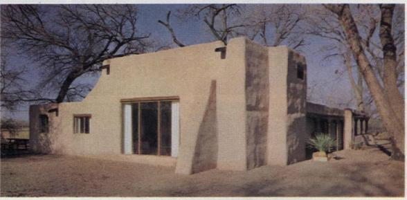
Adobe walls are stucco-covered. Buttress supports the high walls of the living room. Water spouts, or canales, are metal-lined wood. Modern roof was used instead of old type of interlaced branches and adobe.
