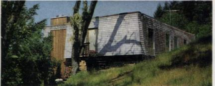
Red cedar shingles virtually cover house, except for chimney enclosure of redwood siding. The stairway leading up from the drive and carport is also made of redwood.
