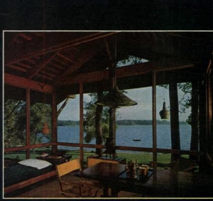
In a house this small, detailing is important since most structural components are exposed. For example, architects Bower and Fradley specified 2x3" nailers on roof so tips of nails would not be seen in living area below.
