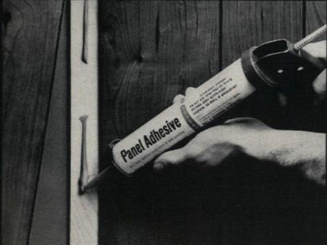
New Weldwood® Panel Adhesive is the successor to hammer and nails, and 50% faster, too, for installing paneling on study or furring. No scratches, no dents, no holes to putty, either.
