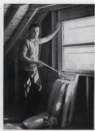
ADDING ON HEATING for new rooms is never a prob-lem with electric heat—it's so easily installed. Here Norman Murchland is insulating his unfinished attic prior to putting in the heating units.
