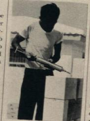
Ribbon of epoxy mortar is applied along block edges.
