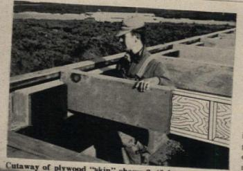
Cutaway of plywood "skin" shows 2x4" frame, stiffener.
