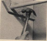
You can make shelf supports for your closets that will do double duty by sawing out a groove in the support to hold the clothes pole.
