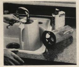
Tank is filled at the sink with warm water. No rinse, low-sudsing household cleaner is added and dissolved in the water. Bag for dirty water fits in top of tank.
