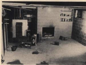
Before. Fireplace wall of unfinished basement shows poured concrete floor and block walls in original state. To provide space around the furnace, a new block wall was brought forward 20 inches. Packaged, premixed concrete was used to cement blocks.
