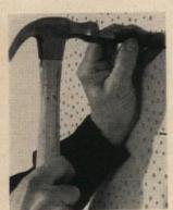
Fasten acoustical tile to furring strips on walls with lath nails, then countersink.
