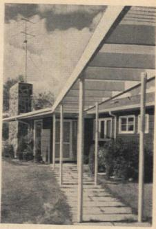
to the family room has a translucent, corrugated plastic roof. Structure for covered walk consists of  $2\frac{1}{2}$ " iron-pipe columns imbedded in concrete piers. Framework for plastic panels is made up of  $2 \times 10$ " fir boards.
