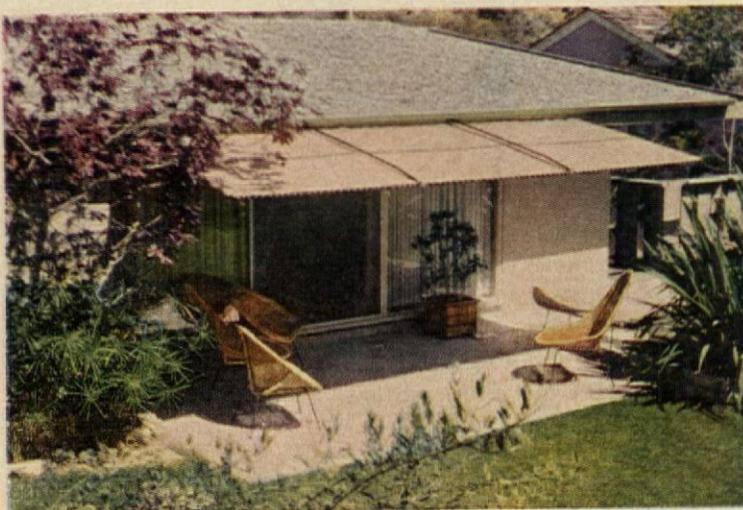
**THIS PATIO SHADE** has pipe-and-flange system that fastens at one end to house fascia board and rests on concrete footings. It can be adapted to most house designs.
