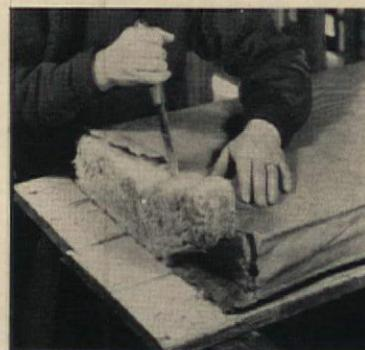
**MAKE A SELVAGE EDGE** for stapling ends of insulation batts to studs, joists, and rafters. Edge is made by cutting wool with sharp knife.
