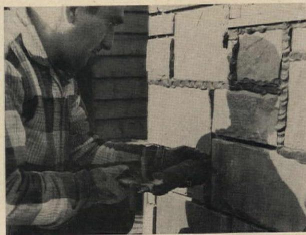
**USE A CALKING GUN** to fill the joints between the stones. Mix one part mortar cement, two parts washed sand with water to a soupy consistency. Screen sand and cement through  $\frac{1}{8}$ " mesh. Fill joints thoroughly.
