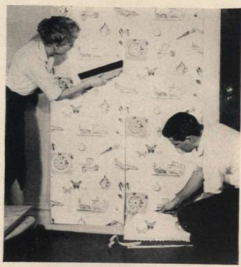
SMOOTHING AND TRIMMING. Smooth out paper with brush, working top to bottom; cut off excess at bottom with razor blade to meet top of baseboard. Paste and hang strips in the order they are cut, sliding edges together with palm to match the pattern.
