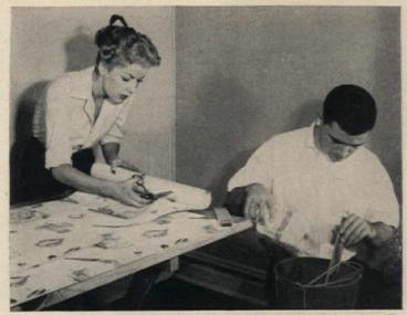
CUTTING AND MATCHING STRIPS. Having measured height of walls, Judy cuts off first strip, allowing extra 6". She then matches pattern exactly with second strip and cuts it off, and so with succeeding strips, each time allowing extra 6". Hank's making wheat paste.
