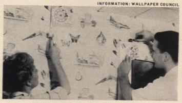
FINISHING TOUCHES. Butted edges are rolled tight. Hank papers over door with short piece matching previous strip and cuts it along door frame. Clean washable paper with sponge, cold water.
