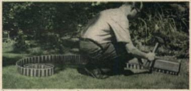
The new corrugated aluminum edging practically eliminates the job of keeping the lawn edged and also makes trimming a good deal easier. The edging comes in rolls and can be cut as needed with tin snips. When the soil is moist, you pound it into the ground with a hammer and block
