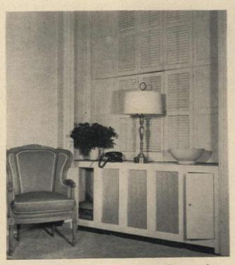
Plus finishing off an end wall in fine style, this cover does a lot more than hide an unsightly radiator core. Both ends are put to work as storage space, one concealing a phone book and telephone, the other a radio. Radiator cover is made of plywood and expanded metal. The reason for the use of metal on the top: to get a maximum heat from the radiator unit.
