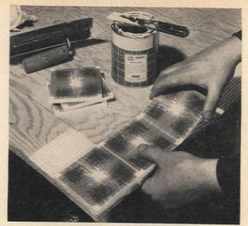
Let's begin: First, mark off corners as shown. Draw a line around the 1/2-inch plywood table top, 41/4 inches in from the edges on all sides so you can use it as a guide for laying the tiles. Place one tile in each corner and continue laying them. These will be in place temporarily, to mark positions with pencil. Remove
