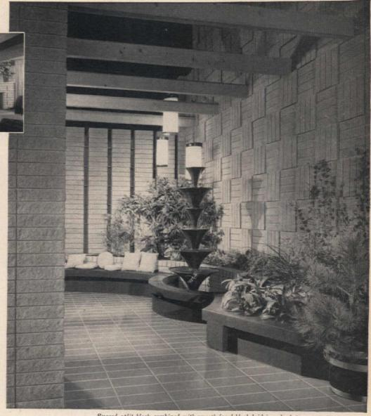
Rugged split block combined with smooth-faced block laid in a basket weave pattern
