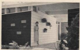
Conventional block with deeply raked horizontal joints
