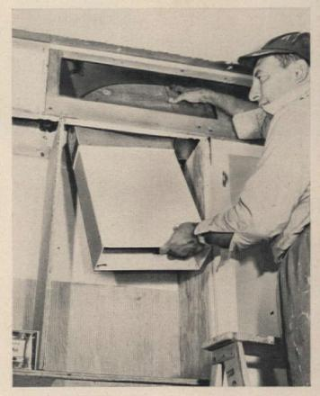
To install piping, remove the facing boards above the cabinets and over the shelves in the recess. Fit and screw together the pipe sections that connect the fan assembly over the stove to the outside exhaust grille. Build a 3/4" plywood frame to house fanblower apparatus; saw opening in bottom to fit intake filter.
