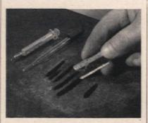
To repair veneer blisters, inject glue into blister with a syringe or medicine dropper. For dropper, first slit blister with razor, Spread glue; weight wood until dry.
