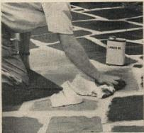
Even off any rough spots in t joints with a cold chisel. A excess mortar on stones can removed with a 10% soluti of muriatic acid and water a plied with a brush. Finally, bring out the color of the ston apply a mixture of half linse oil and half turpentine. Repthis twice yearly for the m imum in attractive appearan
