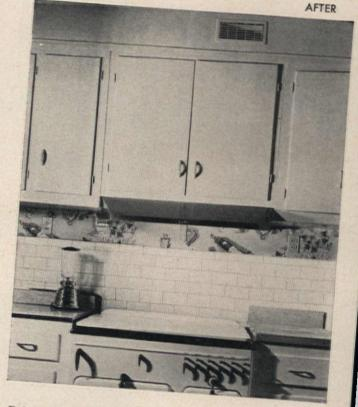
Before the kitchen exhaust fan was installed, recess over the stove was merely waste space—its small shelves did little more than hold bric-a-brac. But a little hard work by the man of the house paid big dividends. Fan kit includes: motor and blower assembly, wall cap and automatic shutter, filters, hood, and onoff switch. You buy standard 9" duct and 34" plywood separately. Booklet you get with kit gives all the specifications.
