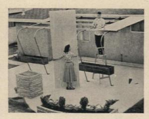
Attach metal brackets to house wall. Thread the tubular steel supports through redwood crossbars. Nail glass-fiber panels in position and seal laps with mastic. Entire patio structure requires no painting and no maintenance.
