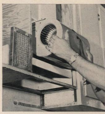
Insert the fan blower under the last section of pipe. The pipe section in front draws in air through the ceiling outlet; pipe in back carries kitchen odors from the stove and ceiling outlets to the outside. Metal air filter (at left), when installed above blower, cleans air brought in through ceiling grille. Filter for
