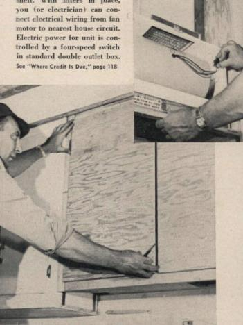
Frame front of recess with 1x2" pine boards, and cut 3/4" fir plywood to size for doors. Fasten doors to framework with semiconcealed hinges, Sand edges of plywood doors smooth, and paint to match other cabinets. Install storage shelves, supported underneath with metal L-brackets, in unused space at left of fan. Install hood by screwing to underside of plywood frame. THE END
