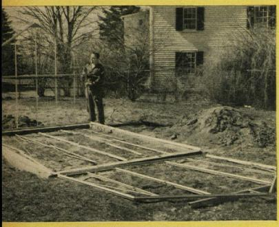
Here's how you start on one of many makes of prefab home greenhouses. First you lay the foundation blocks, then you get the ends assembled.
