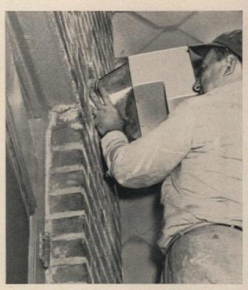
First, break through the exterior wall so that the fan's vent pipe can exhaust kitchen air outside. Because this wall is of brick, the job was particularly difficult. A cold chisel and hammer were used to break through the masonry joints and to remove the bricks. A specially hardened masonry bit with a power drill can also be used. Next fit the elbow and exhaust grille into the opening.
