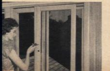
Easy to clean! Gliding Window sash are easy to lift out for cleaning, painting, or changing storm panels. No need to climb ladders. No stretching or straining. Even the large "picture window" sizes lift out in a jiffy!
