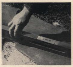
Since the stones may vary in thickness, check the smoothness and slope of your terrace by laying a straight-edged board or level across the stones as you lay them on the tamped sand. CONTINUED ON PAGE 136
