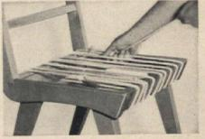
Reassemble chair by coa all dowel and joint surf with a good wood glue. W glue is still wet, use cl or wrap chair with twin soft rope to hold glued faces tightly together glue dries. Let glue set a day or two, then ren rope and replace the
