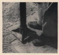
Stake out shape of proposed terrace and remove about 9" of soil so you can provide a base for terrace of 6" of cinders or gravel, and on top of that, 2" of sand. Rake, tamp level.
