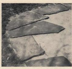
When sand is well compacted, lay out flagstones in the desired pattern and color arrangement. It's best to begin laying stones around the outer edge, then work in toward the center.
