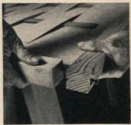
Assemble 2" by 2" frame pieces with 51<sup>1</sup>/<sub>8</sub>" length at top, two 76<sup>1</sup>/<sub>2</sub>" pieces along sides of panel, and 48" length across bottom of panel. Fasten with flat-head wood screws, counterboring screw holes to get professional appearance.
