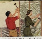
WALLS GO UP FAST! Saw Gold Bond Gypsum Wallboard panels like lumber, or score with knife and snap. If room is upstairs, install Gold Bond TWINSULATION—combines Rock Wool and reflective aluminum foil.
