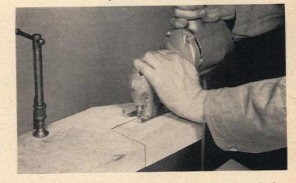
Runners that form the sides of the floor frame are made of 2" by 8" lumber that's notched and beveled at each end. With crossgrain cut already made, saber-saw attachment on the portable unit makes ripping cut, completes notch.
