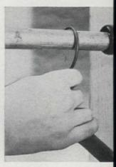
Does your wooden clothe pole sag with heavy coats Take it down and replac it with a similar lengt of iron pipe of the sam diameter. Not only wil the sag disappear, bu you'll also find that th hangers slide easier o the slick surface of iron
