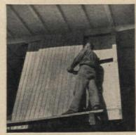
Exterior siding: 4' by 8' sheets texture 1-11 Douglas fir plywood. Siding serves as sheathing, inside walls, weathertight siding.
