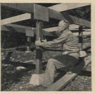
Fasten 4" by 8" girders to posts with 3%" plywood gussets. Over girders go 2" by 8" floor joists and then the 1" plywood flooring.
