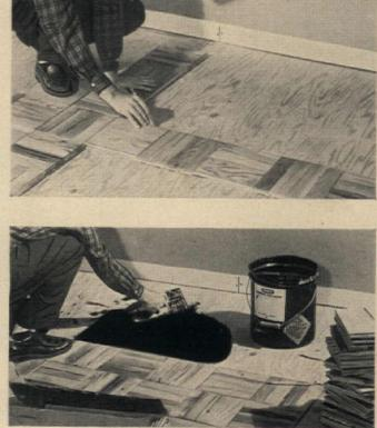
Lay all possible whole blocks on adhesive-covered half of floor. Then shift materials onto completed section, apply adhesive to other half of floor, and proceed as you did on first half. Where blocks fit around pipes, cut hole one inch oversize toward center of room for expansion. Use same clearance at fireplace hearth. CONTINUED ON PAGE 122
