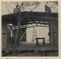
With six bents in place and temporarily braced, fasten the 4" by 4" purlins across bents and then cover 'em with \%" plywood.
