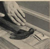
And if you have spilled any adhesive on floor's surface, wipe it off with a turpentined rag. Repaint baseboard and the job is done if you used prefinished blocks. If you used unfinished blocks, finish them with good floor sealer in the color of your choice. Follow the simple directions on the container to get best results. THE END
