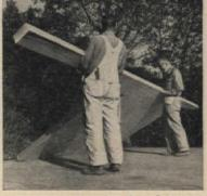
Quick, easy secret of roof over your head is "bent"—one of six used on the house. Build them flat on floor; tip into place.
