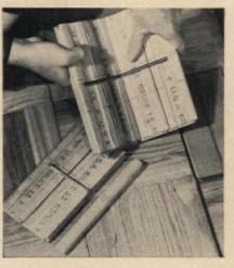
Raise the baseboard to new position so its bottom edge will be about <sup>1</sup>/<sub>4</sub>" above the surface of blocks. Or, if this cannot be done because of location of electrical outlets, trim an equivalent amount off bottom of baseboard. Nail in place. Nail on baseshoe, using a match-cover as temporary shim to provide clearance.
