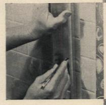
Side pieces are ready-cut and drilled for assembly. Align them vertically with level, mark walls, and then drill. An ordinary ¼" metal drill will do for anything but ceramic tile which requires ¼" drill of tungsten-carbide. Rawl plugs hold screws in wall. Before installing sides, calk wall.
