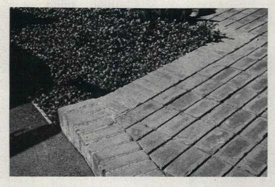
Entrance path is made of bricks laid in sand in a continuous running pattern, held in place by a border of mortared bricks. If hollows form, bricks can be lifted out while you fill in more sand in bed. CONTINUED ON PAGE 150
