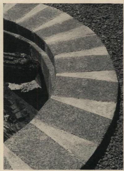
Bricks laid flat around circular firepit are separated by wide mortar joints that help form "radiating" pattern. Designed by Crawshaw and Polleczek. THE END
