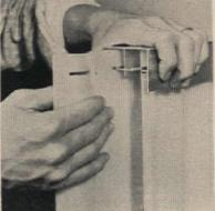
This last step needs an extra pair of hands. Slip one end of top track into place over one side rail, and hold track tilted with doors toward uphill end. Then slide doors downhill while your helper guides their lowered edges into the vinyl-lined bottom track grooves. THE END Look for the man who makes the difference
