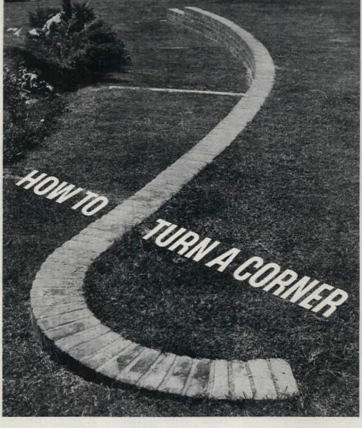
Retaining wall of brick is laid in a fish-hook curve to save grading a lawn that slopes unevenly. Like a dam, wall is curved against thrust of hillside. Footing should be carried below grade at least 18".
