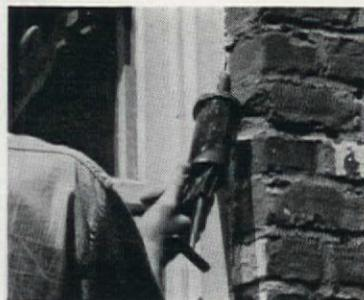
Cracks often appear where different surfaces or materials meet on the outside of a house. Water, dirt, and cold air enter through these cracks and can cause serious damage. Seal the gaps with calking compound, an elastic material that you can apply with putty knife or gun, as shown
