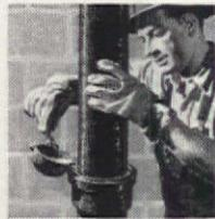
He's pouring molten lead into it—that's what keeps it flexible, yet sealed tight, even if your whole house settles over it. And, before the lead, he rammed oakum into the joint with pile driver force—a force that nonmetallic pipe simply can't take.
