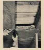
attic roof, the vapor barrier faces down; if you are insulating an enclosed porch floor, the barrier faces up.) (2) Wherever possible, leave a ventilated area between the insulation and the outside wall of the construction (see figure 1). Never force the insulation into the stud space so that it touches the wall, but keep the vapor barrier flush with the inside face of the studs.
