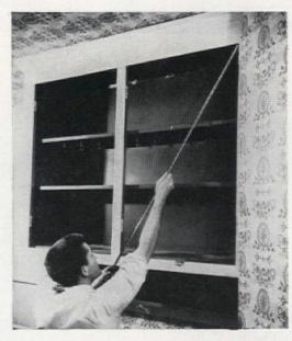
3. If old doors didn't fit well, you'll have to measure the frame openings for the new doors. Check the openings' squareness by comparing the diagonal measurements. If they are equal, opening is square.
