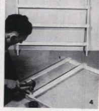
foundation planting from spattering. Needed to make a trellis: A few strips of 1" x 2" lumber (dressed to x 134") cut to convenient lengths; 8-penny galvanized nails; two 3" x 1/4" bolts, preferably with wing nuts for easier handling, to be put through holes bored 21/2" down from the top of uprights. Two such "ladders" make one trellis. THE END
