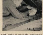
late this area with louvers, at both ends if possible, providing at least one square foot of free inlet and one square foot of free outlet area for every 300 square feet of attic floor area. It is a good idea to cover these vents with screening to keep out insects and rodents, but, if you do, you must double the area of the vent as the screen cuts the flow of air in half.
