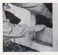
Fig. 3. Board across bottom of doorway on the inside keeps much rain, snow, and dirt from entering, bedding from being pushed out. It can be nailed in place or, if dropped into groove made by nailing cleats to inside of front walls, it can be taken out in summer. Be sure it is free of splinters and rough edges
