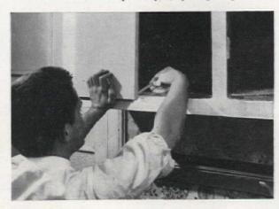
4. Cut the new doors to size for square openings, or ½ inch oversize where openings are cockeyed. Set the oversized door in place, pushed against both the top and side of the opening, and scribe the back of door to get a perfect fit.
