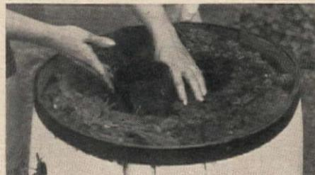
With a spike, punch holes along its length (after filling it with sand to avoid denting it). Set barrel on firm base, put 3" of gravel in bottom, stand pipe in center, and support it while you . . .
