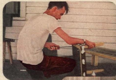
FINISH for walnut veneer surfaces: three coats clear sealer; three coats thinned, one coat regular spar varnish. Other surfaces are sealed, then enameled
