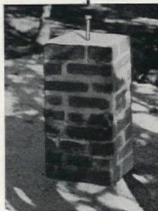
Common brick and mortar make this square pedestal. To hold the table top and bird bath, install a threaded metal rod into the top of the base while the mortar is still wet (to hold the table top on firmly, use a nut). For table top and benches, we suggest thick redwood, cypress, or stout pine boards. The simple benches we show are easy to build, sturdy, and convenient to carry about.
