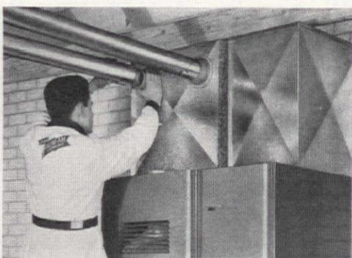
Easiest system to install! Blend-Air is completely pre-engineered for fast installation. 3½-inch round ducts fit in walls between studs, save costly remodeling. Coleman's compact furnaces and cooling units fit in basement, attic, closet, utility room or under-floor crawlspace.
