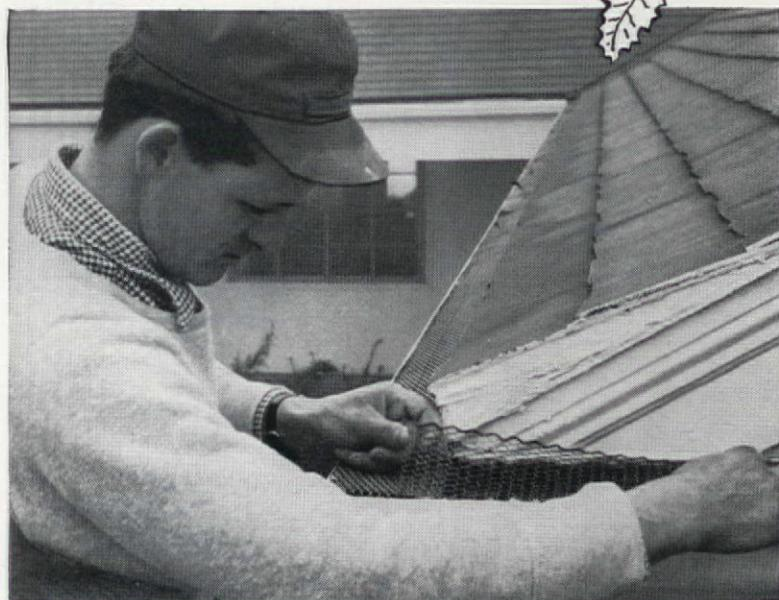
Tired of semi-annual gutter cleaning? Then build these leaf-proofers. First clean gutters. Then cut 1/3" galvanized hardware cloth into strips an inch wider than gutters. For wooden gutter, nail screen to one edge. For metal gutters, staple screen to roof under first row of shingles, or bend up small lip along screen edge and staple to side of house. Overlap all joints
