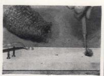
Steel wool packed in the old hole will also tighten loose screws
