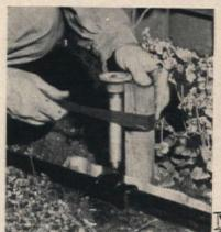
Semirigid pipe sprinkling system is first laid out roughly on surface of ground, tees and metal sprinkler heads attached and staked up, connected to water line and, after letting joint cement set 30 minutes, tested for ground coverage. Pipe and sprinkler heads can then be buried to proper depth
