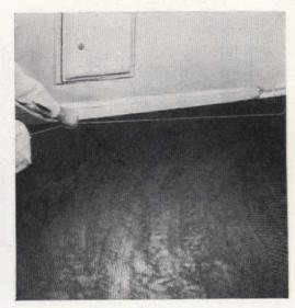
8. Since marking tile may pick up adhesive, keep it off the finished floor. Scribe marked tiles deeply with a linoleum knife. Snap tiles in two along scribed line. Sand edges smooth. Fit tiles into place
