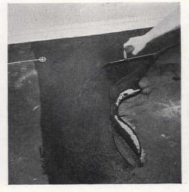
7. To fit borders, use one tile (B) for all marking. Lay a tile of border color (A) on last row (C) of installed tiles. Align edges. Place marking tile (B) on top of A. Push B flush against wall. Scribe A along edge of B
