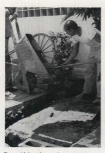
To avoid frost-heave, footings were put in at the outside edges of the new room. They should extend below the frost line and be poured concrete or built up out of masonry block
