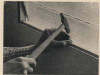
Cut two quarter-round moldings to fit across the width of the opening. Nail one strip on the inside bottom of the frame so the bottom louver rests against it when closed and one at the top on the outside. Position moldings carefully so top and bottom louvers are weathertight
