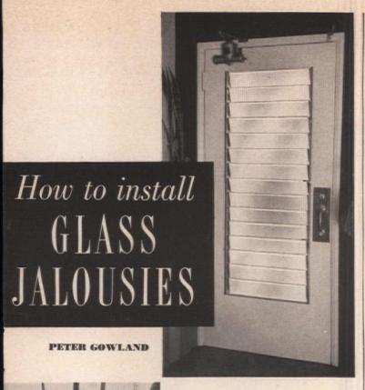
If you have sturdy glass- or woodpaneled exterior doors, you can install adjustable glass jalousies in those doors to increase both light and ventilation. Remove the molding from around the panels, and then remove the panels themselves. If panels are of glass, remove putty and glazier's points. Inside face of opening has wood molding that must be removed as jalousie mechanism must be mounted on flat surface
