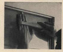
To avoid hitting the glass with the hammer when attaching moldings, slide the hammer along the back of your hand as shown, or use a strip of wood to guide the hammer when nailing. The two molding strips, if carefully fitted, will make the unit efficiently weathertight against the wind and the rain
