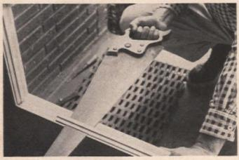
The inside molding is usually an integral part of the door and must be cut off with a saw or a chisel. Plane or sand the surface smooth, give the exposed wood a coat of preservative, and apply a coat of primer to protect the surface before proceeding further
