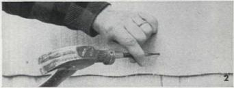
Brush and wash asbestos cement shingles as described above. Then check for loose shingles. These should be renailed at top edge. To avoid splitting, drill a hole through the shingles (both layers) and drive nail with a nail set completely through outer layer
