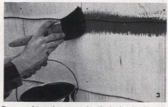
To prevent drips and runs, paint the siding's edges first, being careful to get full coverage of the under side. Use the brush flat, not edgewise, even when painting the under edge of the siding. Painting with the edge of the brush will result in a streaky job and will cause the brush to wear unevenly. Do the edges of an area about three feet square at one time before filling in the area between the edges
