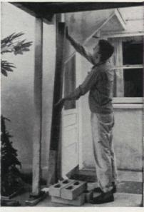
One of the posts had to be removed to allow the new masonry block wall to be built. Before taking out the post, a 2 x 4 was cut to size and used to shore up the roof beam
