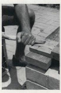
A lap joint was made where boards meet. Lay one board on other, flush with the end, and saw halfway through it. Use a heavy chisel to finish the cut. Repeat cut on other board
