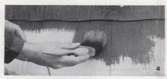
In painting the flat surfaces, first brush the paint out and into the fine crevices of the shingles. Then finish up with broad sweeping strokes, using tips of bristles and lifting brush gradually at end of stroke to feather out the laps
