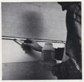
5. Secure panels to wall with 8-in. finishing nails countersunk below wood surface. Locate wall studding by sounding, and mark location on lower part of wall. Nails should be driven into studding, not plaster and lath alone. Coat rabbet with wood glue
