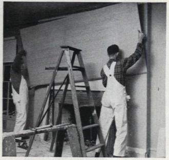
3. Cut ¾-in plywood to size of fireplace. Place sections on wall horizontally to eliminate vertical joint centered directly over fireplace opening. Meeting edges of panels are rabbeted to produce half-lap joint, with rabbets ¾ in. deep, ¾ in. wide
