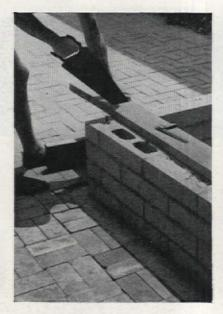
Base sill for the windows was made from 2 x 6 redwood boards. Note the bolts projecting from the wall. These special anchor bolts were set in during construction of the wall
