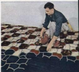
Low installation costs for Armstrong's Flagst Asphalt Tile are due to this unique "grid-unit" of struction. Square "mortar" grids fit together precision-cut, shaped tiles drop into position.
