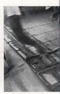
Three parts sand were mixed with one part cement and very little water, and worked between bricks. This dry mix requires sprinkling with water every 12 hours for two days
