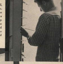
The louvers are cut from glass 3/16 in. thick. You can do it yourself, but for the amount of accurate cutting involved, a "pro" may be advisable. When cut right to size, the louvers slide into place with ease
