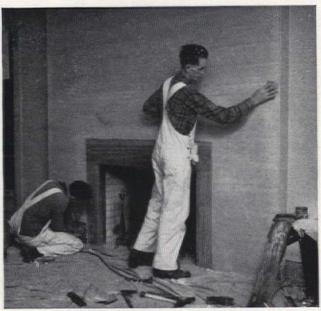
8. If you use unfinished plywood, sand down horizontal joint and sand whole panel lightly. Avoid sanding through top veneer of plywood. Apply stain desired—walnut was used here—and wax. Exposed edges may be covered with hardwood strips
