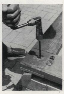
With an expansion bit, holes big enough for washers were drilled part way through top board, just deep enough so washer and nut would not project above the surface of sill
