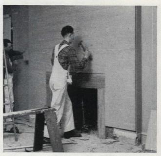
7. As standard plywood panels are 4 ft. wide, two will take care of average 8-ft. high wall. If slight gap remains at bottom, as in this case, it can be covered by a simple baseboard. If larger gap results from high ceiling, use small filler piece of plywood
