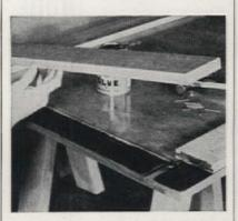
Complete job by laying the four non-rabbeted pieces onto glued surface. Place as shown, so that joints will overlap. Nail the two frames together, set the nails and fill the holes. When the glue is dry, the door is ready to be hung
