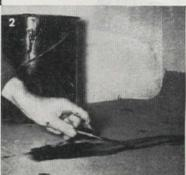
2. Make a permanent, vapor-sealed floor by applying a layer of asphalt crawl-space covering or 55-lb. roll roofing over entire ground area. Run material about 2-in. up walls, lap it 2-in. at the seams, and seal the latter well with roofing cement
