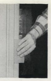
2. When dry, put wedge under door, reset longer screws. If door rubs frame lightly, rub paraffin block along surfaces where friction occurs
