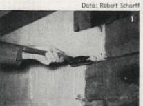
Earthen floors in basements and crawl spaces often encourage excessive water vapor which pervades the house to stain ceilings, mildew wallpaper, and commit other evils. First, level ground, fill holes, tamp. Coat walls with white cement paint
