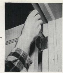
1. If door sticks, check hinges for loose screws. If screws won't hold, glue wood plugs in holes, or fill with plastic wood, let dry thoroughly
