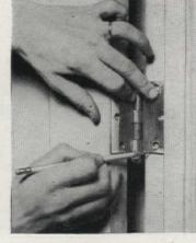
9. Binding of a heavy door can often be relieved by adding third hinge. Open hinge, mark and cut mortise. Align door and attach MORE PICTURES ON PAGE 91
