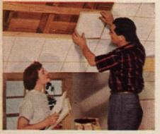
The J-M Ceiling Panels went up easily and quickly using a handy stapling tool. (We could have used nails.) The Lightning Joint worked like magic hiding all staples and lining up the panels, snugly and evenly
