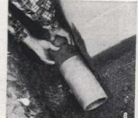
10. Good circulation of air is essential. You need about 2 sq. ft. of opening for each 100 linear ft. of foundation. If you're lacking screened vents above the grade level, it's a simple matter to install some in each of the sidewalls
