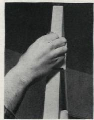
4. If hinges are tight but door sticks on latch side, sand spot where binding occurs, using medium-coarse sandpaper, then fine
