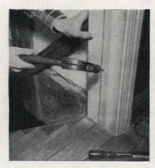
8. If the door sticks against the stop, carefully pry up stop with a chisel and reset it slightly away from the door to provide additional clearance
