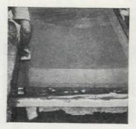
finished with an edging tool. the surface is finished. Pile it with straw, burlap, cotton mats, or impervious paper, and keep it well saturated for at least 72 hours. Proper curing adds to the strength and durability of the sidewalk-so don't shirk
