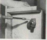
Cut dados in the side pieces for the top and bottom, and also for the shelves. Bottom shelf should be set far enough up from floor level to take a caster which helps the hinges support the weight of the door when it is loaded. Caster should be attached on outside edge of shelf on latch side
