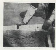
After preliminary leveling with shovel, fresh concrete is struck off-as shown here, with a template or strike board. Use same concrete mix for the full depth of the sidewalk
