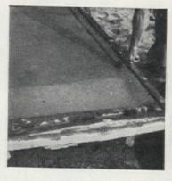
A few hours after the concrete has been poured it should be stiff, but still workable. Finish the surface with a wood float. This smooths the surface yet leaves it rough enough to furnish a sure footing. The man in this picture is edging the sidewalk so it will have a groove along the sides
