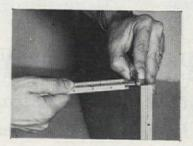
Side panels are fastened to center section with piano hinges. Hinges should be set ¼ in. beyond edge of plywood so that they will come flush with face of mirror. Install hinges to side panels and drill holes for hinge screw in center section. Use long wood screws to give ample support
