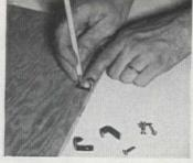
Mirrors are fastened to plywood backing with U-shaped brackets sold at hardware stores. Make recess in edges of plywood so that brackets will fit flush with surface. Install two brackets at top and bottom, one at side
