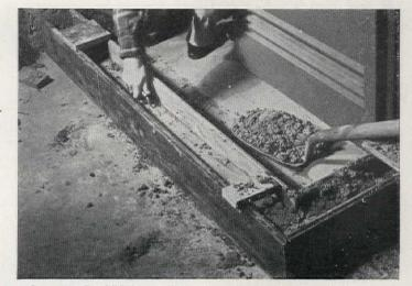
Concrete should be poured into forms before the grout is dry. Use a mixture of one part Portland cement, two parts sand, and three parts gravel. Mix the cement with the sand, and then add the gravel. When the three are thoroughly mixed, add water and continue to mix until you have a workable plastic. So that it is well compacted, the concrete should be tamped and worked as it is placed in the forms
