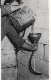
To treat area around footings in homes where there are masonry-block foundation walls, drill holes two or three feet above the floor so that the solution can be poured into the voids in the block and seep down to footings. Place holes at all vertical joints. A funnel and a short piece of hose are used to pour the solution into the center of the masonry walls "If you can paint a room, you can insulate your attic with KIMSUL\*
