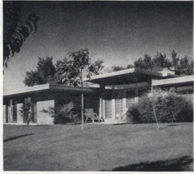
The modern look of the Hornbein home is dramatically evident in this view of the exterior. Note the generous overhang of the flat roof that shelters the small terrace. Note, too, the modernized version of French doors that open into the living room. A separate Honeywell thermostat assures wintertime comfort in the area behind these doors by compensating for heat lost through the large glass area.
