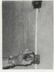
The anchor nails should be set about 12" apart along the chalk lines. Put the anchor nail in place and then twist it around a little so that there will be an even coating of adh sive under the entire plate about 1/16" or so in thickness
