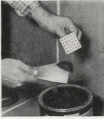
Mark off vertical chalk lines on the wall where the furring is to be placed. For most jobs, the lines should be 24" apart. Apply a small amount of the adhesive—about the size of a walnut—to the back of each anchor nail. The nails can be used on floors as well as walls
