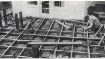
With the patio area leveled and its pattern laid out, 2" x 4" redwood headers were held in place by being nailed to firmly driven stakes. The four posts at the left are the framework of a redwood plant box beside which two broad steps enter the patio
