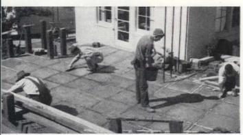
as the concrete is poured between the redwood strips. Note the four pipe supports for the future trumpet-vine trellis, the plant box, left open at the bottom for drainage, and, in the foreground, the top of the new, higher redwood retaining wall
