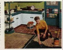
With half the floor installed, Mrs. Loock spreads Kentile Adhesive to cover remaining half. Then it's simply a matter of putting tiles in place until entire floor is completed.
