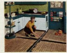
Here Mrs. Loock finds the center of the floor. Next, she'll spread Kentile Adhesive over half the floor before laying the tiles in place.
