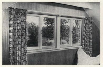
Here are close-ups of windows which do so much for rooms on page 57. One is a 5'6" x 4'6" sliding unit; the other a pair of sliding units combined to give a 3'6" x 7'6" opening. They cross-ventilate so well that this attic actually cools off faster than downstairs on hot days
