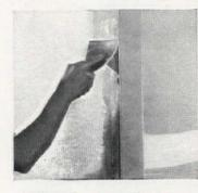
Additional coats of adhesive are applied over tape portion of bead so it is completely concealed. Don't move position of bead during this process
