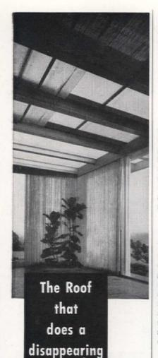
The sky's the limit for this unusual room which makes fullest use of its surroundings to create an effect of breathtaking beauty. Sturdy Smooth Rough Wire Glass has been used to form a roof of light. and the panels can be rolled back to create an open air porch. These versatile skylights permit effective control of sunlight and breezes ... help accomplish an atmosphere of full liveability.
