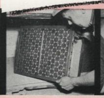
Filters on forced-warm-air heating systems should be cleaned or replaced at the start of the heating season. While you're at it, brush down the blades of the blower and remove dirt from filter housing
