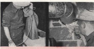
Dirty chimney (a serious fire hazard) can be cleaned with a burlap bag weighted with stone or metal, filled with sawdust or excelsior. Dirt and soot can be removed through clean-out door at chimney base Check to be sure that stovepipe from furnace does not extend into chimney flu as this will spoil chimney draft.
