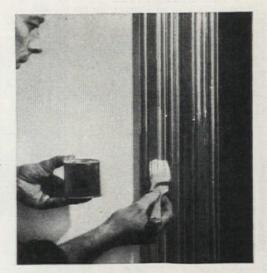
Let sealer dry: 4 hours for alcohol-base; 24 hours in warm, dry weather for aluminum. Then apply enamel undercoat which makes flat base, good under enamel. Tint undercoat to approximately final shade. If first sanding smoothed woodwork and there is no serious dust between sealer and undercoat, you need not sand again before enameling. For semi-gloss instead of high gloss, add some undercoat to final enamel coat
