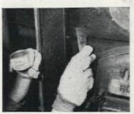
Small cracks in cast-iron heating equipment can be patched by first cutting out opening with small file. Pack in iron cement. The heat will fuse the cement into a solid mass
