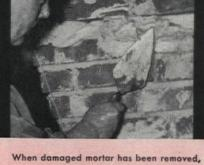
When damaged mortar has been removed clean out the opening, wet down edges of surrounding masonry, and pack joint with mortar—one part Portland cement and three parts sand, or readymixed mortar sold at hardware stores
