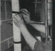
Pipe insulation is slit down one side so it can be slipped around pipe and secured with metal bands. Return line on two-pipe steam system requires no insulation as this would delay the steam condensing into water
