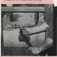
Dirt and compound are removed when boiler is cold by opening drain valve at base and flushing inside of boiler with a garden hose held to various boiler openings after fittings have been removed
