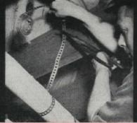
Noises in the heating system are often caused by pipes that are not properly supported, have sagged at some point, or don't slant down from radiator to boiler. Use a level and see that they have the proper pitch
