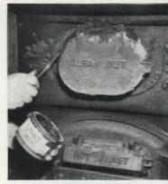
Openings in furnace must be tight for plant to operate efficiently. Clean-out doors and similar openings should be sealed at the start of the season with furnace cement
