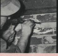
After you have found the leaks in the chimney, cut out the cracks so they can be patched. Cutting out can be done with hammer and cold chisel, but be careful not to damage the surrounding bricks and mortar joints
