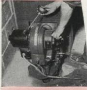
Be sure oil-burner motor is cleaned and properly oiled. If manufacturer's oiling instructions are not handy, fill oil cups with \$10 motor oil. Refill cups one hour after first filling.
