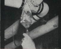
Breaks in pipe insulation or areas around valves and fittings should be patched with asbestos cement. Wet down surrounding insulation, mix dry asbestos cement with water and apply to damaged area with a trowel
