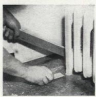
A pounding steam radiator can usually be silenced if small blocks of wood are put under the legs at the opposite end from the pipe connection. This allows the water to drain out of the radiator
