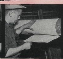
Efficiency of warm-air system can be increased if air ducts are wrapped with asbestos paper. Two layers will do, and the paper can be held in place with lengths of wire. Inside of ducts should be cleaned by vacuuming
