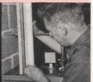
Be sure that all warm-air ducts slant up from the furnace to the registers. If they have sagged so they have a downward slope, they will not deliver heat properly. Wire or metal bands Hot-water pipes and steam lines should be incased with asbestos air-cell insulation to prevent heat loss. Insulation comes in 36" lengths to fit standard-size pipes. It can be cut easily with a knife
