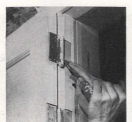
The mortises exposed when hinges are moved can be patched by cutting snugly fitting strips of wood, and fastening these into place with glue. When the glue is hard, the patch may be trimmed down to exact size with a plane or sandpaper
