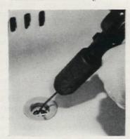
For clearing badly clogged pipes, use a piece of flexible cable gripped in a drill chuck
