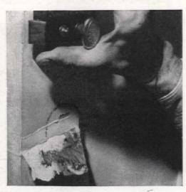
Holes and marks in the wood can be filled in with a wood filler. For large patches, a second application of filler may be required to compensate for shrinkage. When the filler is dry, sand the surface down with sandpaper
