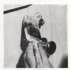
Coats of primer-sealer, enamel undercoater, and one coat of enamel should be applied to the new work. Then give the entire door a single coat of enamel. If you paint the lock, keep the key in it so that paint won't get in
