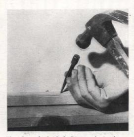
The job may be finished off in a professional manner if molding is applied on both sides of both halves of the door, where panels meet the sill and the reinforcing strip. Molding is fastened in place with small nails or brads
