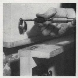
The two halves of the door are locked together with a dead-bolt lock installed in two holes bored in the upper half of the door. Main lock on lower half allows either the lower half or the entire door assembly to be locked closed
