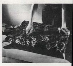
Place plastic on cemented surface. Smooth over cemented area with small squeegee, working out center. Lift up the rest of the plastic, sponge cem on wood, replace plastic, squeegee smooth. Ceme sides, smooth. Trim corners. Turn edges under
