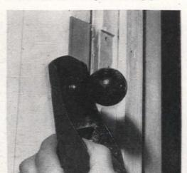
Door gets two cuts,  $1\frac{1}{2}$ " apart. A sill of  $3\frac{3}{4}$ " stock,  $3\frac{1}{2}$ " wide, is attached to bottom half, and a reinforcing strip of  $3\frac{3}{4}$ " stock is attached to top half. First, make cut along cut-off line. Then attach sill. Lay reinforcing strip on sill and use it to scribe second cut-line on top half
